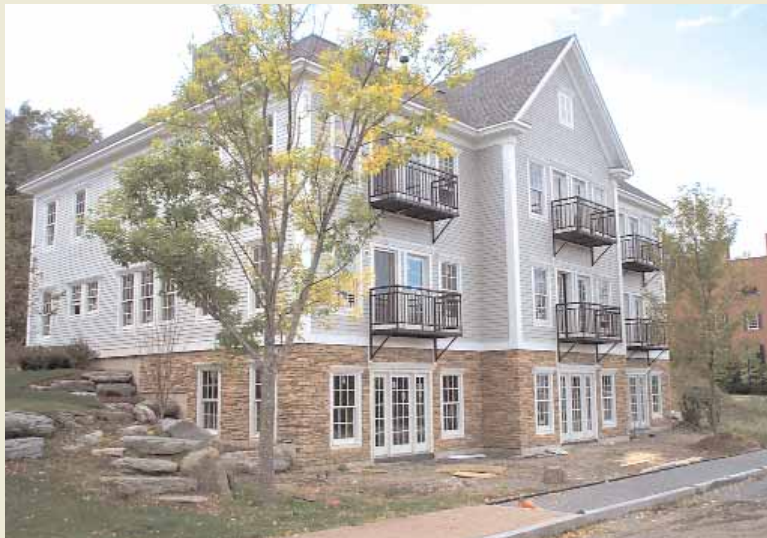
Depot Street Condominiums, under construction
